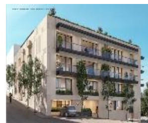
40-42 Ardittou str., Mets – Reconstruction of building Athens
