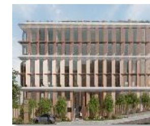
199 Kifisias Ave. Marousi – Reconstruction of existing office building Athens
