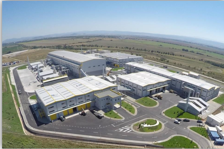
Mechanical Biological Treatment plant, Sofia, Bulgaria
