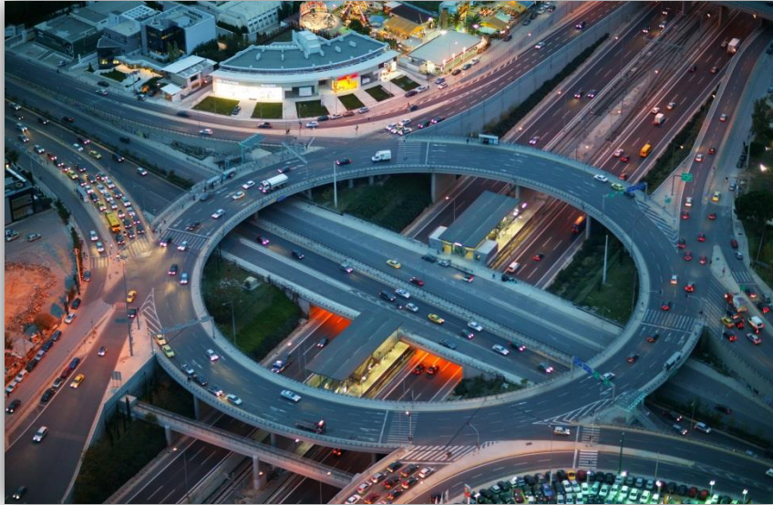
Attiki Odos, Athens, Greece
